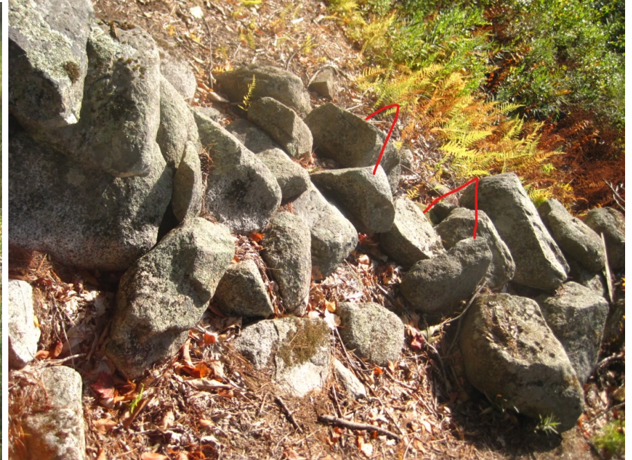
2020 granite split by the weight of equipment, see red lines
