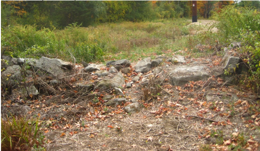
2020 WP-8 (west wall) crushed, was 2 feet tall
