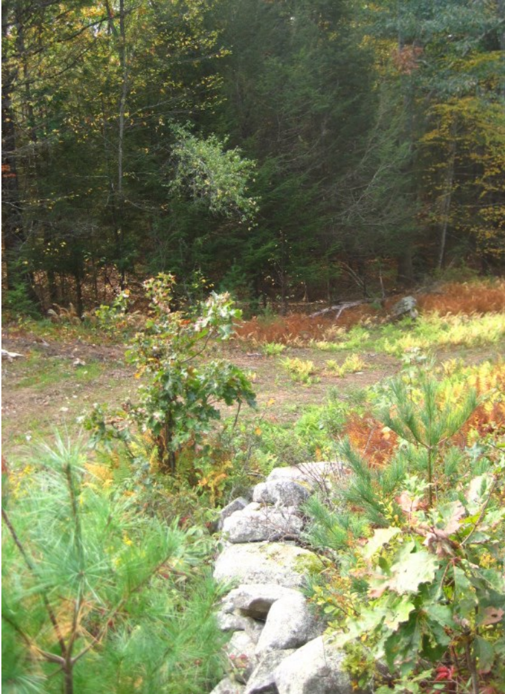
2020 south breach, was 9 ft, now 57 feet wide
